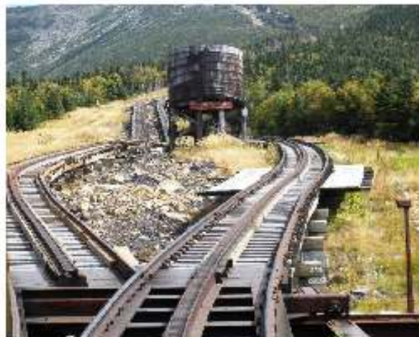
Water tower and switch needed for two way traffic
